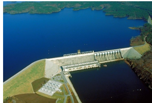
Υδατοταμιευτήρας USACE Richard B Russell Dam and Lake, Source: http://en.wikipedia.org/wiki/Richard_B_Russell_Dam#mediaviewer/File:USACE_Richard_B_Russell_Dam_and_Lake.jpg Jonas N. Jordan, U.S. Army Corps of Engineers - U.S. Army Corps of Engineers Digital Visual Library Public Domain1994
