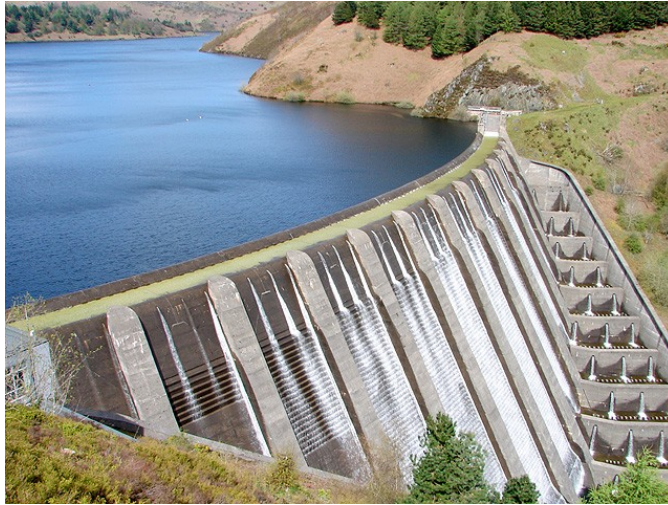
Clywedog Dam and Llyn Clywedog Reservoir.
