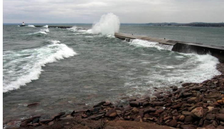
Breakwater at Presque Isle Park Marquette
